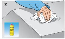
Use thinner to thoroughly clean the surface to be insulated. Insulation is not recommended where there is incrustation or other flaws which could prevent the sheeting from sticking perfectly.
